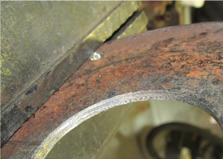
**Figure 10, Cleaned up Orifice Plate**
